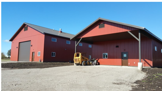
NWARC Pesticide Storage & Shop buildings
