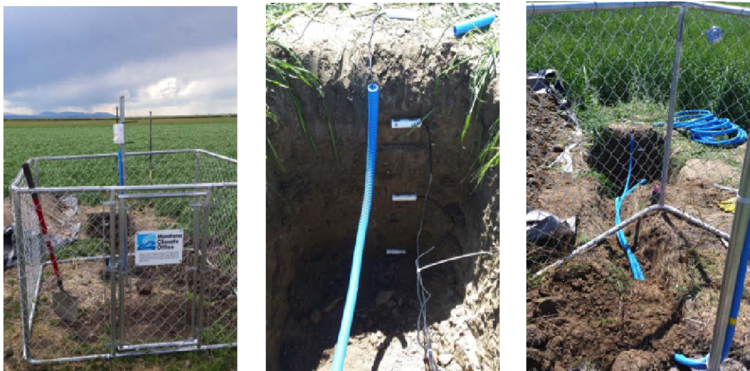
Figure 2: An example station installation with soil moisture, soil water electrical conductivity, and soil temperature measurements at 3", 8", 20", and 36" depths.
