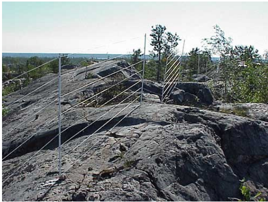
This installation involved blasting holes into the rock to insert the fence posts.
