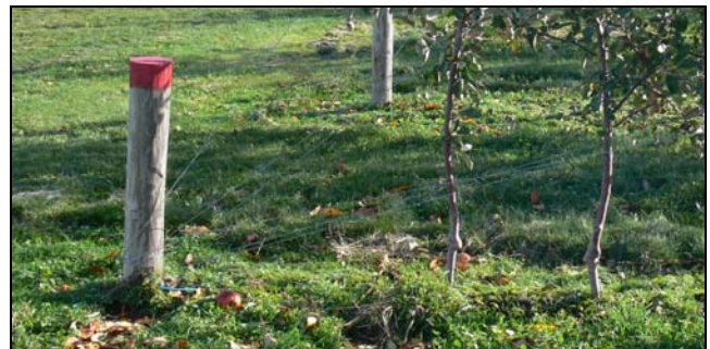
Figure 6. This post-type anchor has been pounded vertically, but if it was installed with about a 10^{\circ} lean against the pull (in the same direction as the angled end post) it would strengthen the entire assembly. (Photo: Hugh Fraser)
