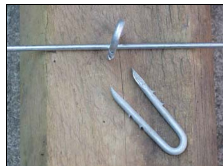
Figure 12. Staples with slashed end points like the one on the left in Figure 11 should be positioned at 20-30° off vertical to the 'right' over the wire (1 o'clock) as shown above. This helps reduce wood splitting and forces the staple legs to rotate away from the flat slash face of the staple. Staples with slashes like the one on the right in Figure 11 should be installed at 20-30° off vertical, to the 'left' (11 o'clock) over the trellis wire. Fortunately, when you buy a box of staples, they are all alike. (Photo: Hugh Fraser)
