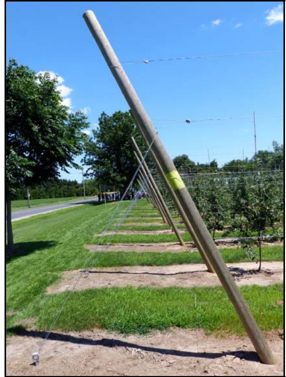
Figure 5. Angled-brace, end-of-row anchor system. Note the 60^{\circ} angles between the post, wire and ground, forming an equilateral triangle for maximum strength. The end post should be pounded, or vibrated in at least 3-4 ft into undisturbed soil. This installation uses a shorter tie-back wire 7 ft off the ground, instead of from the top of the post, to minimize space. This trellis uses 16 ft posts with 3.75 ft in ground to accommodate future hail nets. This requires longer and heavier anchors. (Photo: Hugh Fraser)
