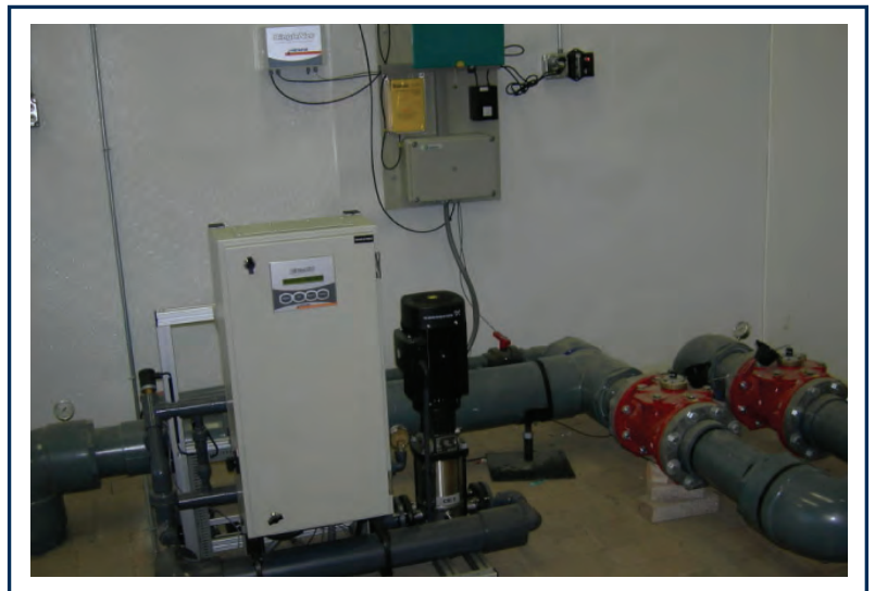
FIGURE 4. Fertilizer injection system
