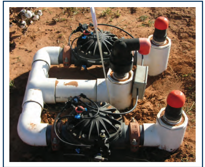
FIGURE 3. Example of a field installation of pressure regulating valves and air release vents
