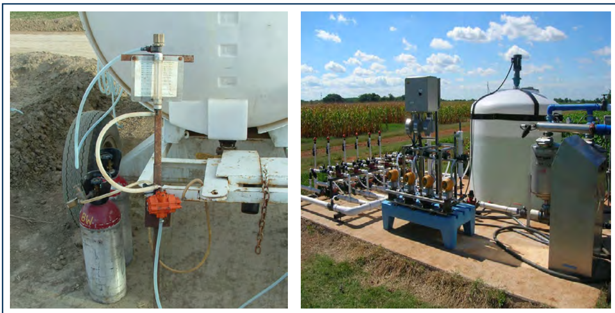
FIGURE 13 (left) FIGURE 14 (right). Examples of fertilizer injection systems
